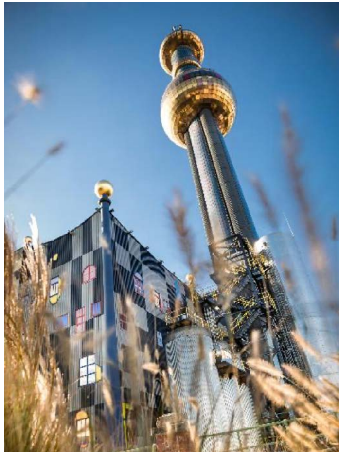
The municipal solid waste- (MSW)-to-energy plant in Vienna operated by Wien Energie converts 260,000 tonnes of MSW per year to heat and electricity for the capital of Austria (exterior design by Friedensreich Hundertwasser) (Photo credit: Wien Energie/Ludwig Schedl)
