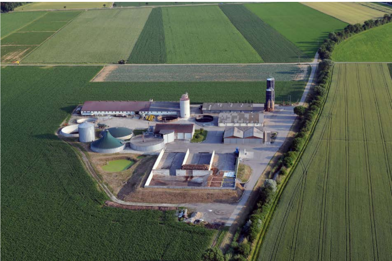
Biogas plant integrated into an agricultural setting in Austria (Photo credit: ROHKRAFT/Karl Pfiel)
