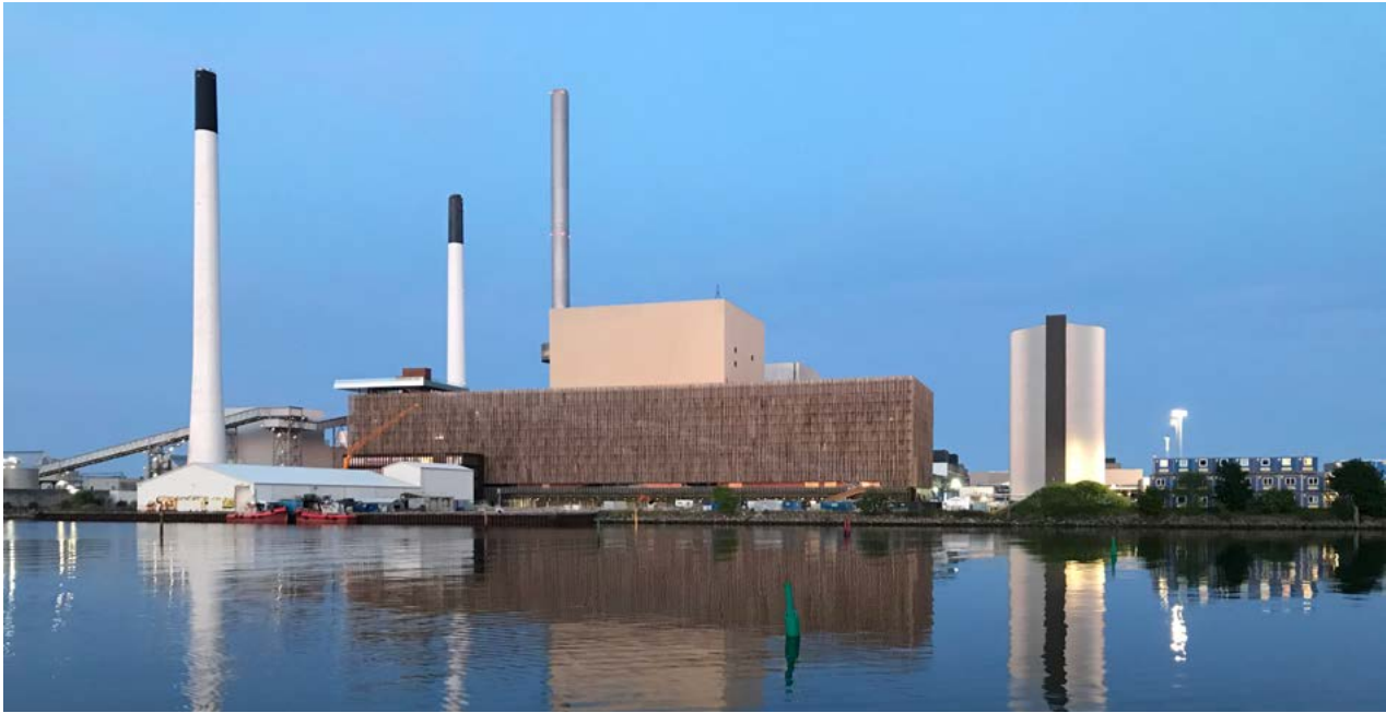
Bio4 at Amagerværket, run by the Greater Copenhagen Utility (HOFOR) is one of the largest biomass CHP (cogeneration) plants worldwide with a wood chip fuel capacity of 500 MW, providing heat and power to the city of Copenhagen (Denmark). (Photo credit: Morten Tony Hansen)
