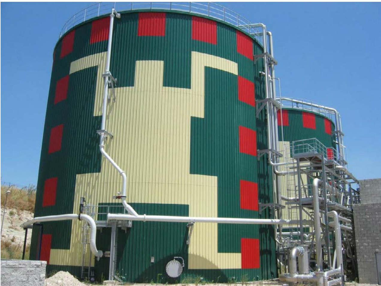
Biogas plant treating organic waste (Pinto, Spain) (Photo credit: University of Natural Resources and Life Sciences, Vienna/IFA Tulln)
