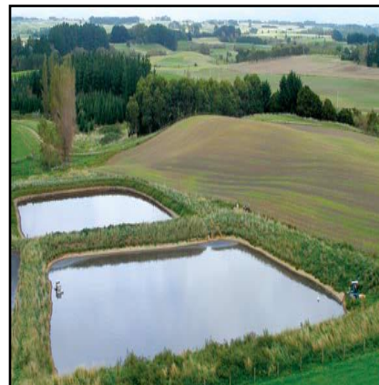
Ponds used for effluent disposal can provide the raw material for a biogas system. Covers also help to reduce odour.
