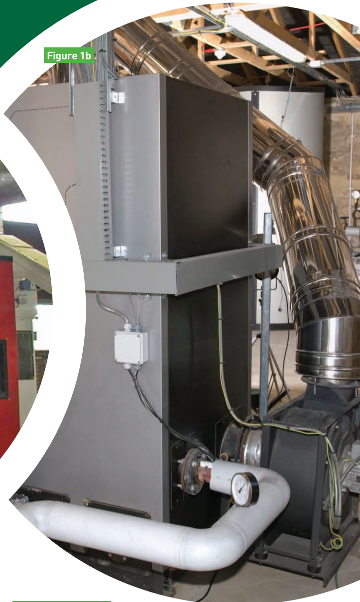
Figure 1 (a) and (b) Medium scale commercial boilers (Forestry Commission).
