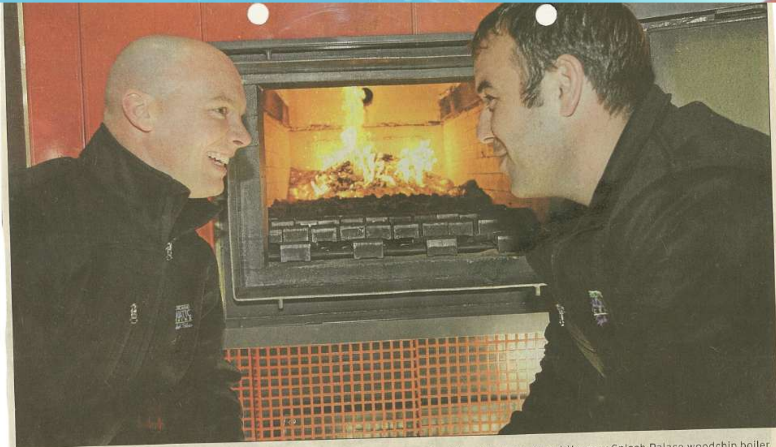
Good result: Aquatic services manager Pete Thompson, left, and plant supervisor Steve Cook check out the new Splash Palace woodchip boiler. Photo: ROBYN EDIE/FAIRFAX NZ 626740885
