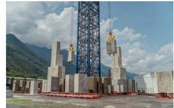
Figure 4: Working energy vault gravitational storage system
